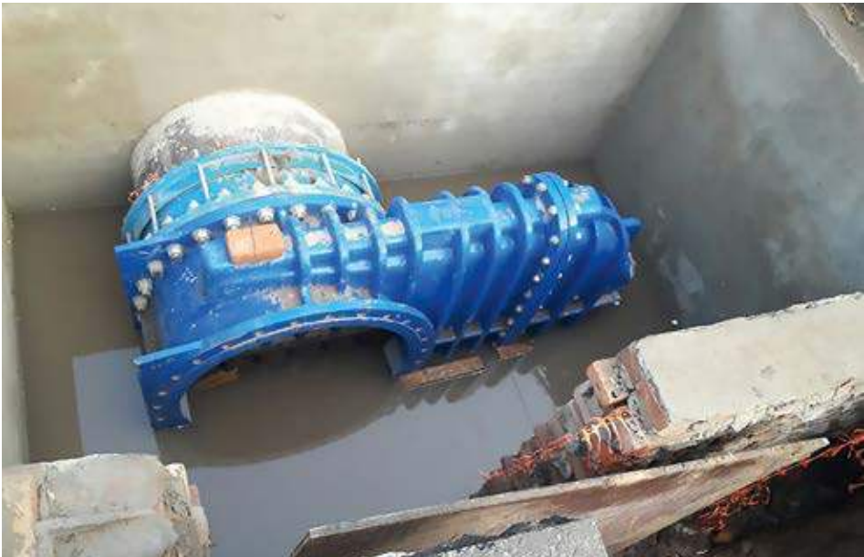
One of the faulty gate valves that caused an emergency in the province of Santa Fe
