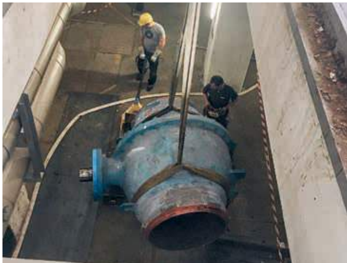
Removing a KHSVI ball valve after 25 years of use under difficult conditions
