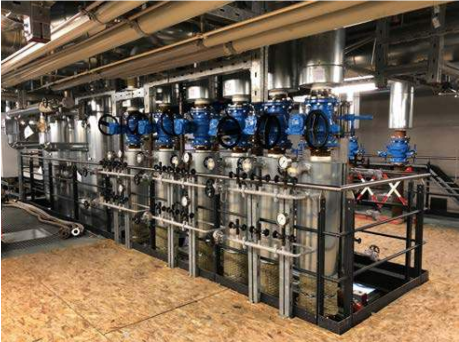
A row of DN 150 KLINGER Ballostar KHI ball valves installed at Erdwärme Grünwald
