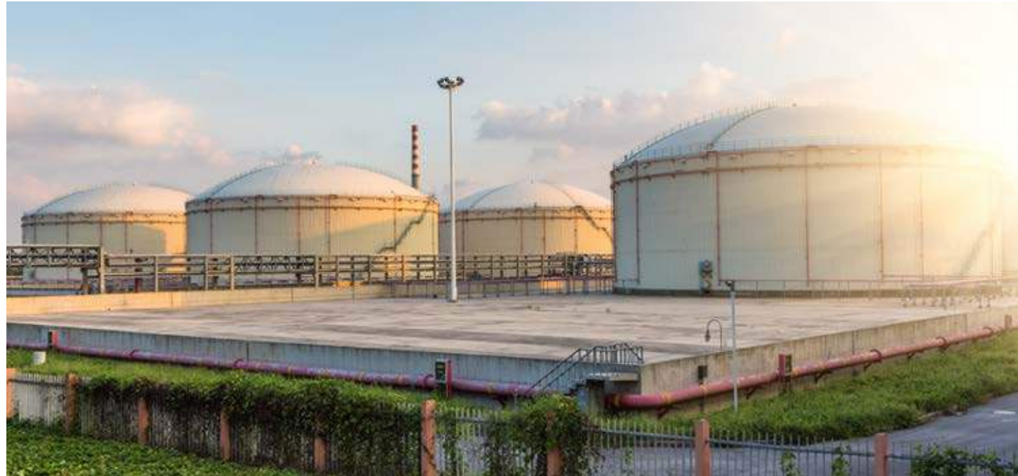
Biogas facilities help generate electricity and heat
