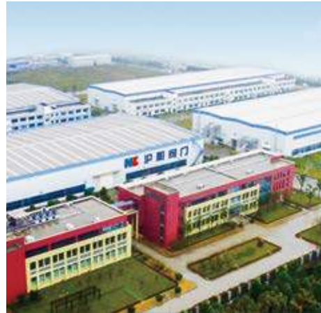
Hudong valve factory in Shanghai, China.
