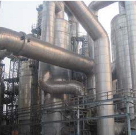
A typical sulfuric acid plant in Zambia
