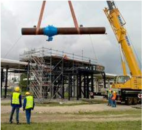
Transportation of a 12 t district heating pipe including a KLINGER Ballostar® KHSVI
